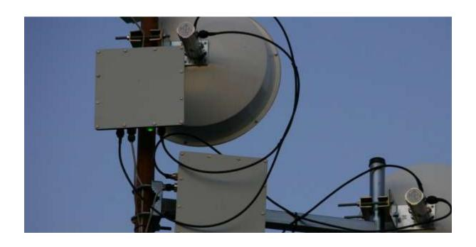
InfiNet Wireless solutions were used in the deployment of a fully upgraded, wireless CCTV system.
